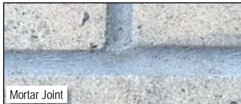
Tooled mortar joints are best suited for masonry-bound trim items such as belt courses, lintels, window surrounds, date stones, inscription blocks, quoins, keystones and similar applications. Rake and point the mortar joints rather than full-bed setting and finishing in one operation. See Technical Bulletin #44 on Pointing.
