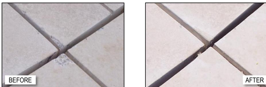
Climatic conditions must be taken into consideration before the repair is to commence. Do not repair stone in freezing weather or if a freeze is anticipated within 24 hours. On hot sunny days repairs should be done during the morning hours where the cast stone is shaded or at temperatures less than 90 degrees Fahrenheit. Repairs should be covered with a damp cloth and plastic sheet to prevent the water from evaporating before the cement has hydrated.
