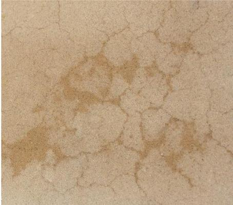
Crazing has been a concern since concrete has been in existence. The appearance of small cracks on the surface, especially when filled with water or dirt, can be alarming since it is assumed that the fissures are running through the entire cross section the concrete. But in general, crazing does not affect the structural integrity of the concrete and should not by itself be cause for rejection. All cement based products and many natural stones are susceptible to crazing.
